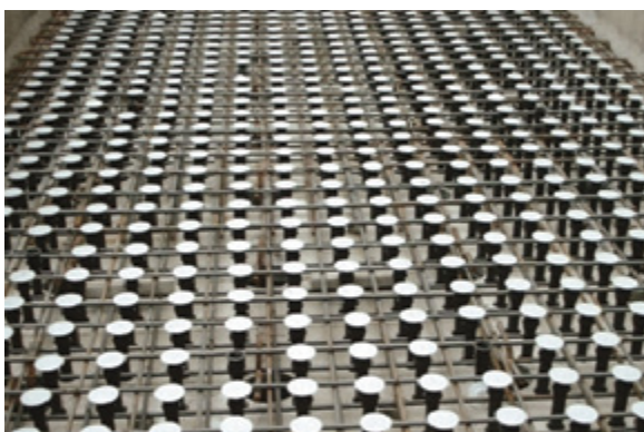
Installed threaded sleeves and protection caps
