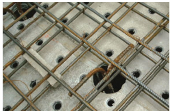
Steel reinforcement showing connecting steel within column form
