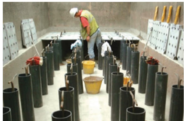
Column forms, cut to size and leveled
